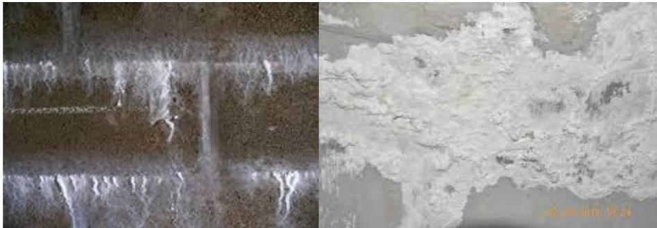
Efflorescence is not to be confused with laitance, which is the appearance of a loose, powdery deposit of cement powder and sand fines on the surface of concrete. Laitance is caused by excess water in the concrete mix, by poor concrete curing practice (i.e. failure to apply wet hessian, wet sand or a curing membrane or, at the very least, plastic sheet over the wet concrete and thus allowing the concrete surface to dry out prematurely) and by over-trowelling.
